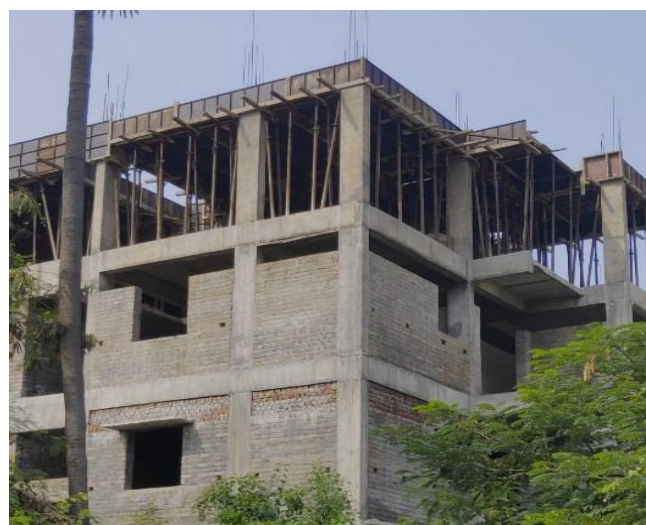
Fig. 3. Current Construction practice on RC framed structure
