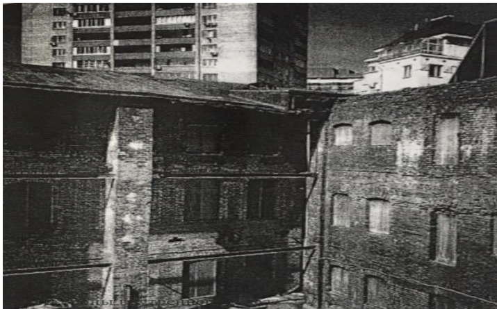
Fig. 1. General view of the brickwork of the external walls.
