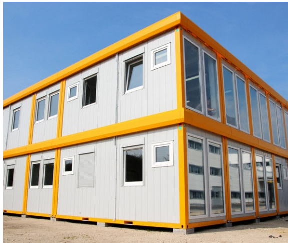
Fig. 4. Quickly erecting modular building.
