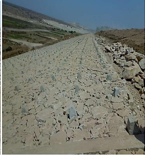
Fig.4: rip rap with hand picked stones at U/S (upstream side)
