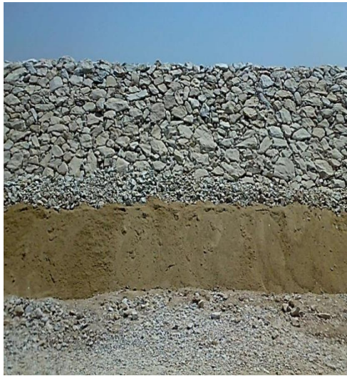
Fig.3: Sand drain with rockfill above @ toe drain
