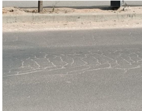
Figure 5. Measuring of Cracks
