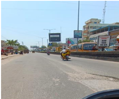
Figure 4. Mesurement of Potholes
