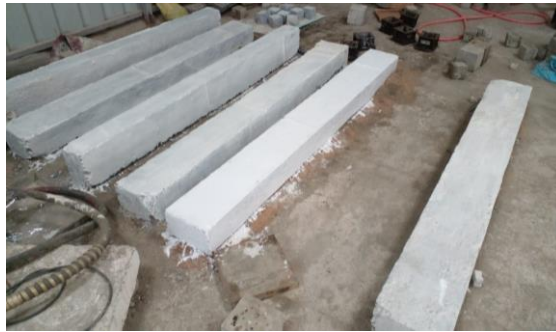
Figure 5. Beam Reinforcement and casted beams
