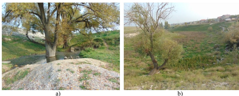
Fig. 3. Violations recorded at reservoirs 13 and 14 located in the upstream of the Abdalka river: a) flooding of the dam lower reaches of the pond 13; b) view of the pond 14.
