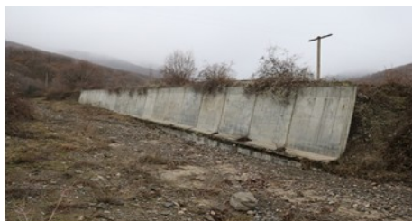
Fig. 2. The current state of the cantilever retaining wall p. Gromovka.
