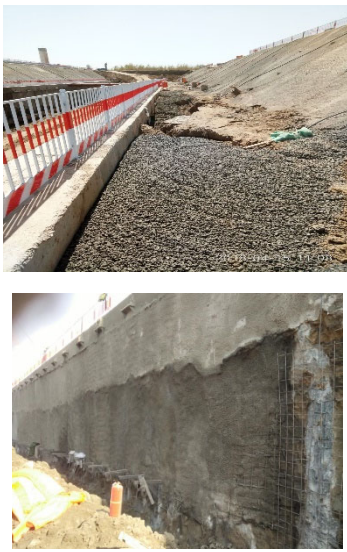
Figure 22. Anti-leakage measures on the inside of the foundation pit
