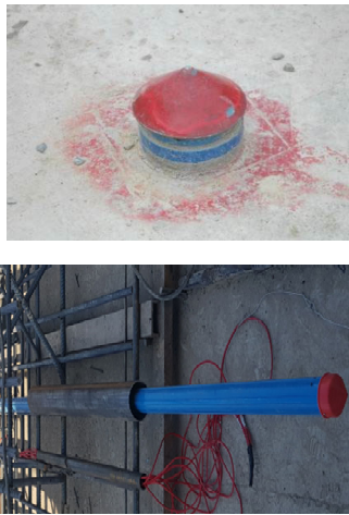
Figure 11. Protection measures for the inclined tube
