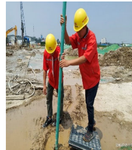
Figure 3. PVC water level tube
