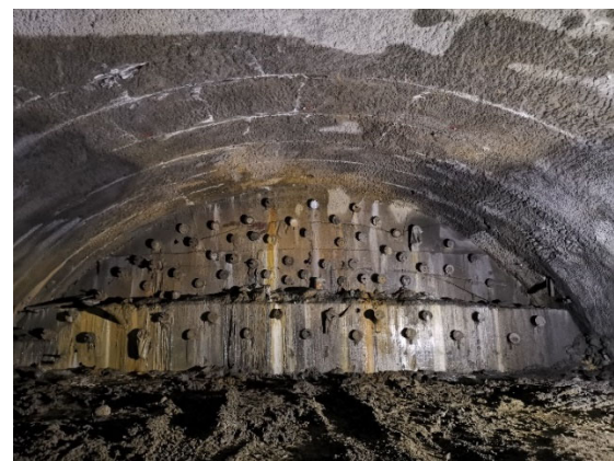
Figure 3: Curtain grouting
