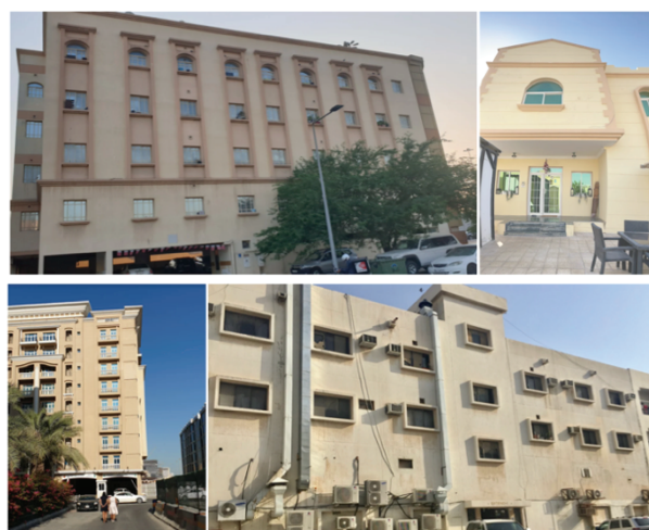
Fig. 1. Typical buildings surveyed
