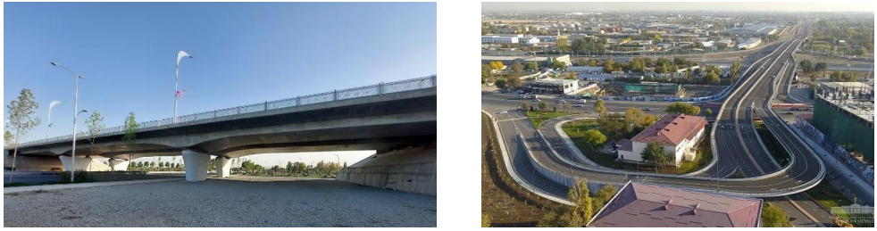
Fig. 1. Modern continuous (monolithic) reinforced concrete overpasses built in Samarkand.
