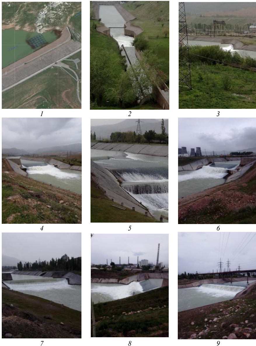
Fig. 3. Bypass channel with water-cutting energy absorbers of Angrenskaya mine
