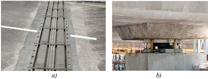
Fig. 5. Modern bridge devices used in monolithic bridge building: a is expansion joints; b is seismic protection bearing parts
