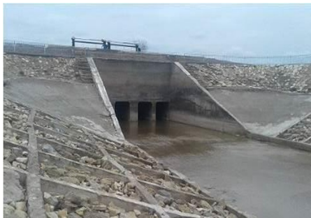
a) View of the structure from the downstream
