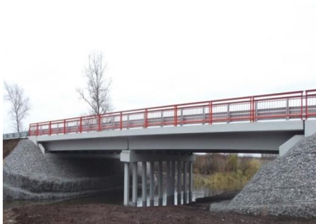
Fig. 1. Reinforced concrete road beam bridge
