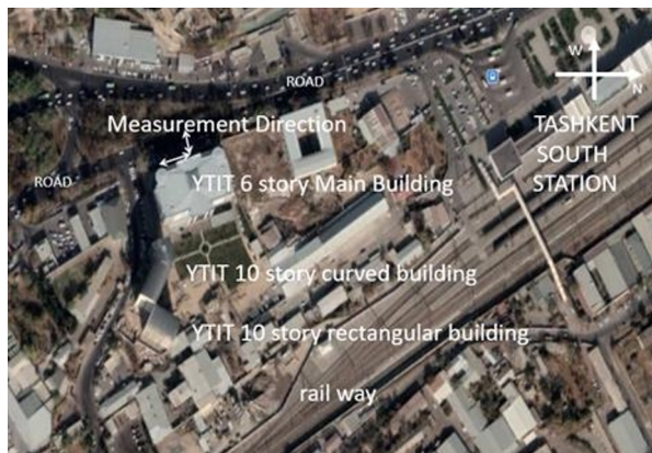
Fig. 3. YTIT building site location
