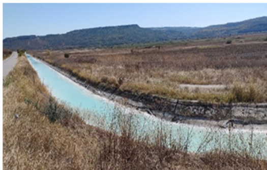
Fig. 8. Sewage drainage channel of the Padina tailings pond
