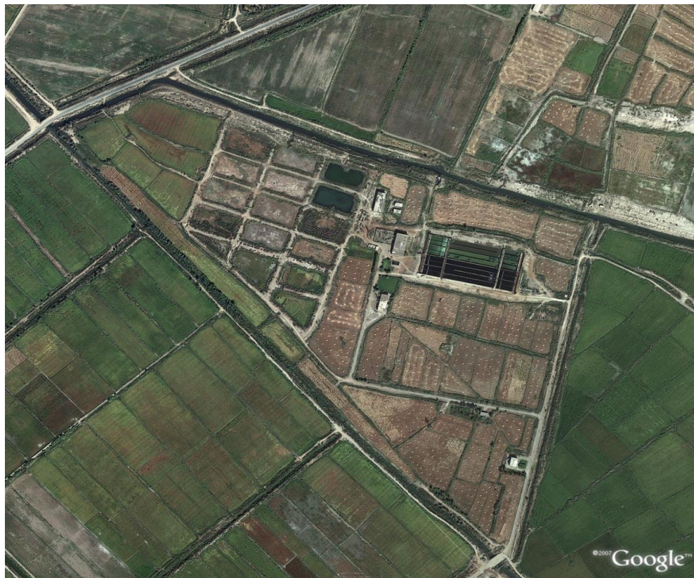
Figure 1. Aerial photo of the biological ponds of “Khorezm water supply” Ltd.
