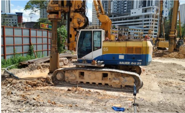
(a) Piling Activity
