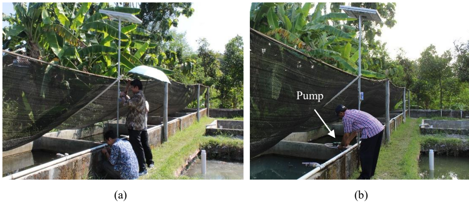
Fig. 5. Installation of SPS: (a) solar module and pole, (b) water pump
