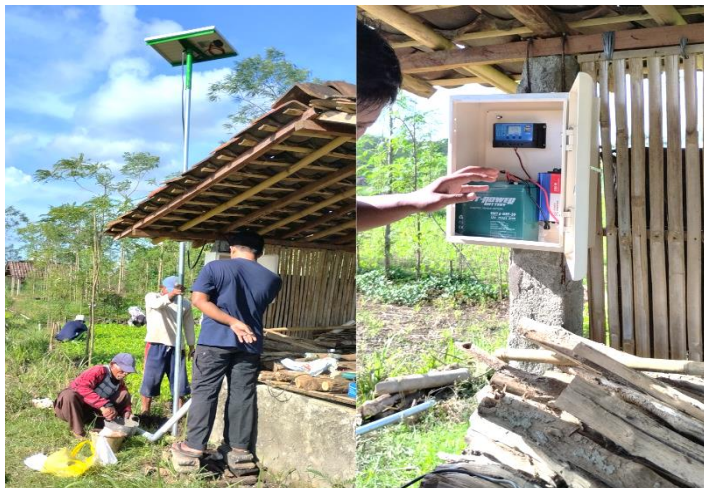
Fig. 4. Installation of the solar-powered hut (Pragak village).
