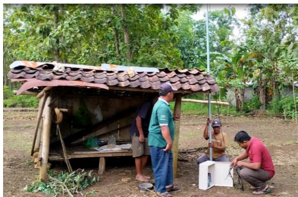
Fig. 5. Installation of the solar-powered hut (West Nitikan village)
