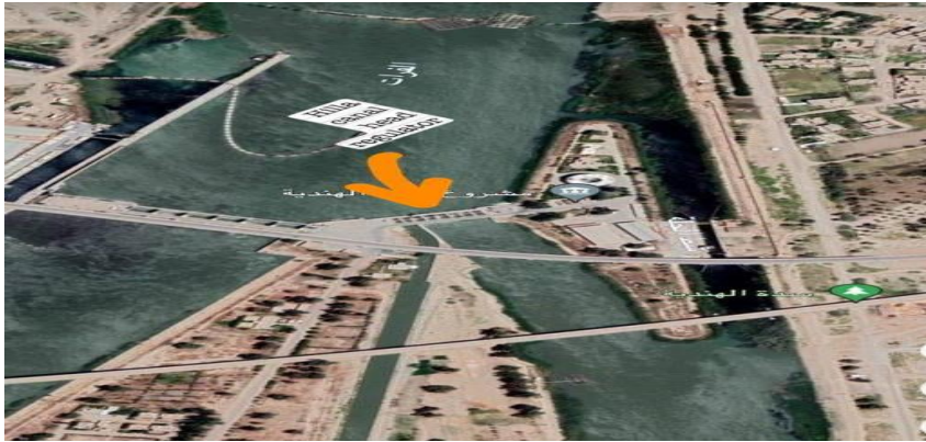
Figure 1: Hillah Canal Main Regulator
