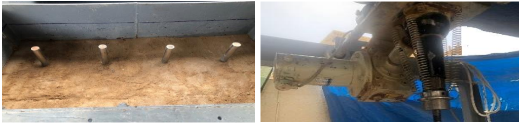
Figure 3: Piles embedded in soil and mechanical jack.
