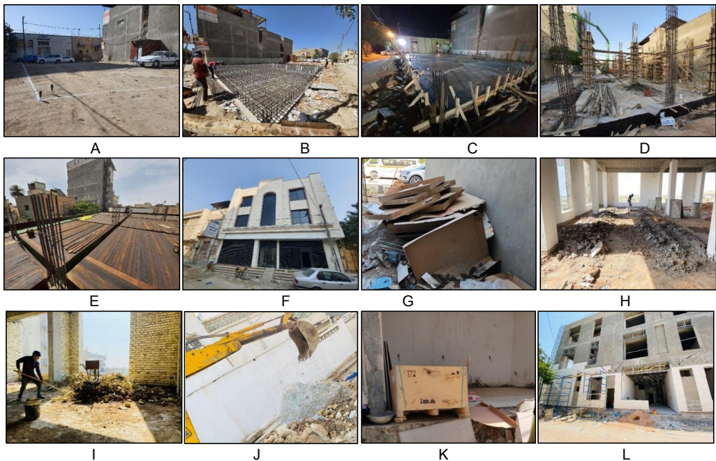
Figure 2: Construction stages and waste generated during building construction.
