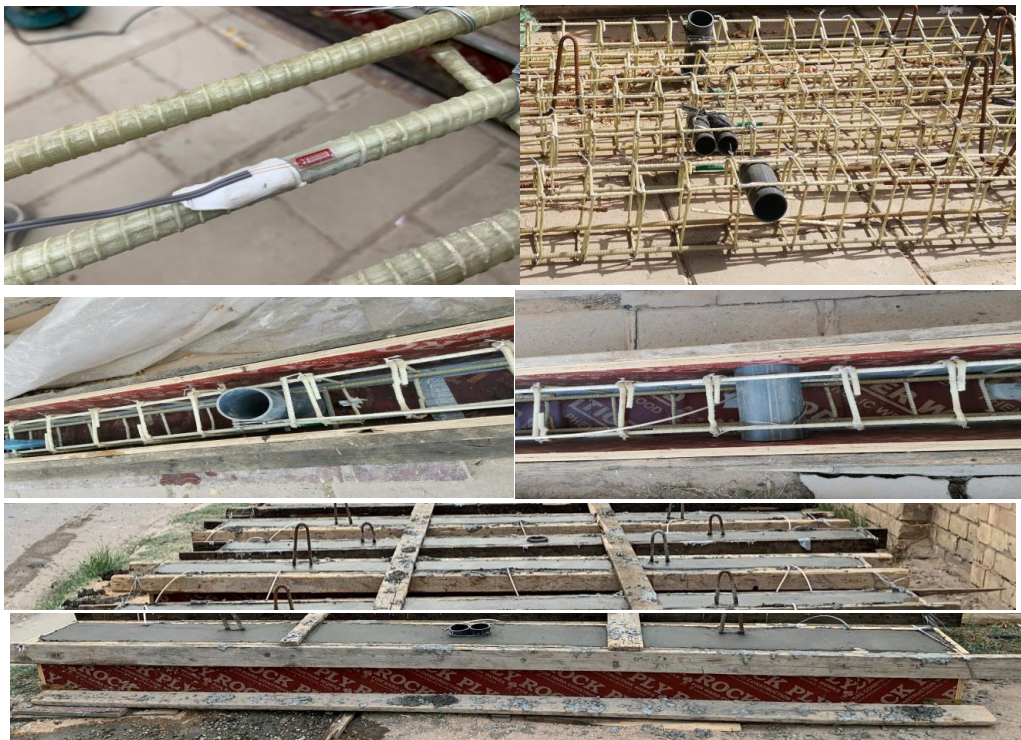
Figure 2: Reinforcing and casting of the tested beams.
