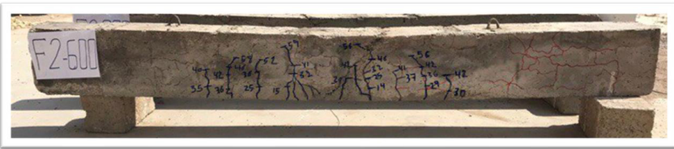
Figure 18: Cracks pattern for the specimen (F2-600).
