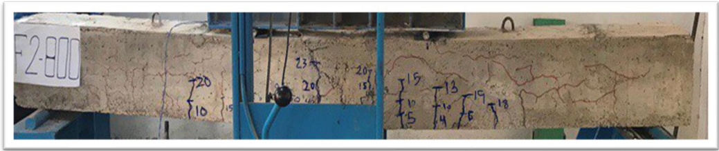
Figure 20: Cracks pattern for the specimen (F2-800).
