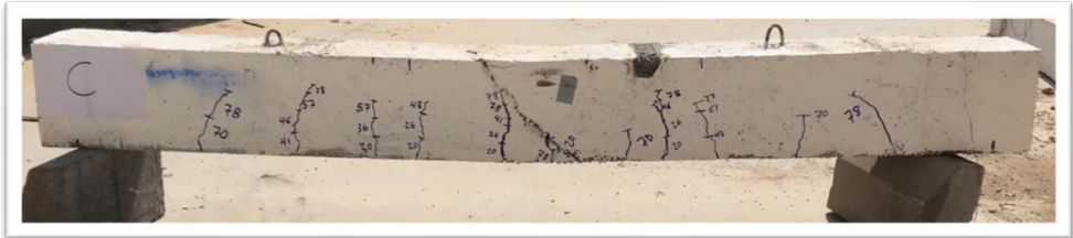
Figure 16: Cracks pattern for specimen (C).
