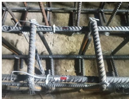
Figure 3: Strain gauges installed on the tensile reinforcement.
