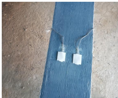
Figure 4: Strain gauges installed on (CFRP) sheets
