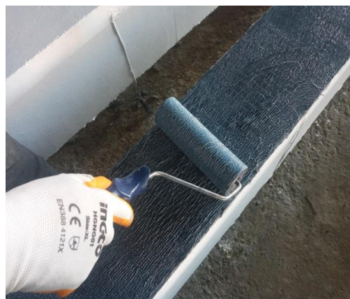
Figure 2: Adhering (CFRP) sheets.
