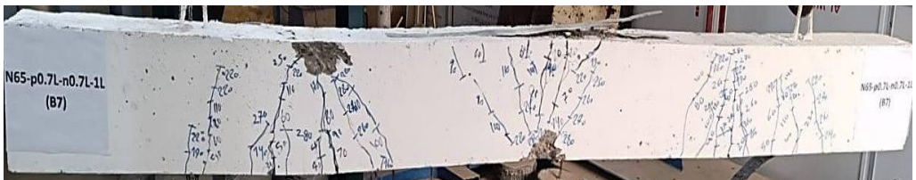
Figure 9: Map of cracks for N65-p0.7L-n0.7L-1L.
