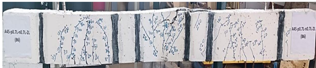
Figure 8: Map of cracks for A45-p0.7L-n0.7L-2L.
