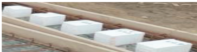
Figure 9: Styropor pieces used for constructing the opening.
