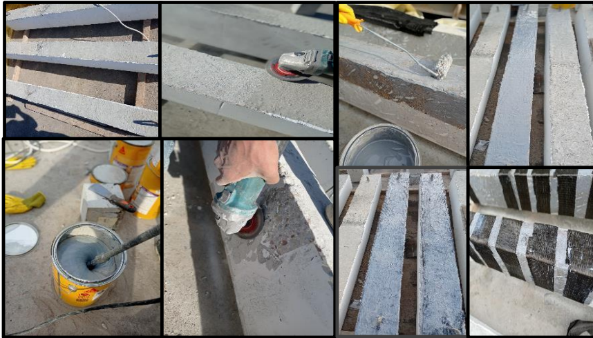
Figure 4: The application of CFRP Sheet.
