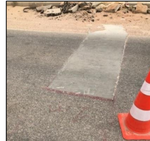
Figure 5: In-situ section after opening the road lane.
