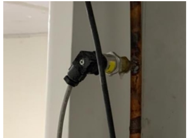
Fig. 4. The Gems Sensors 3100 series are used to measure refrigerant pressure intrusively.
