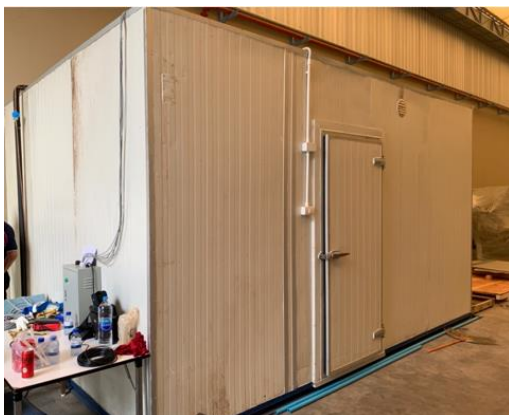
Fig. 2. Test chamber constituted from 4-inch PU panels.
