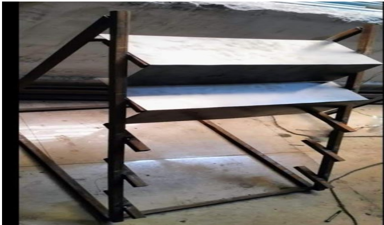
Fig.7. Fabrication of stair case (step -2)
