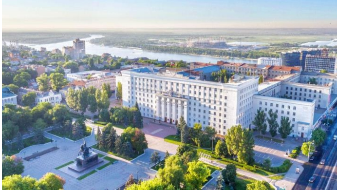
Fig. 3. Presents the building of the Government of the Rostov Region with the surrounding landscape.
