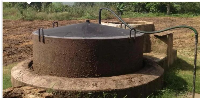
Fig. 5. Floating Drum Digester
