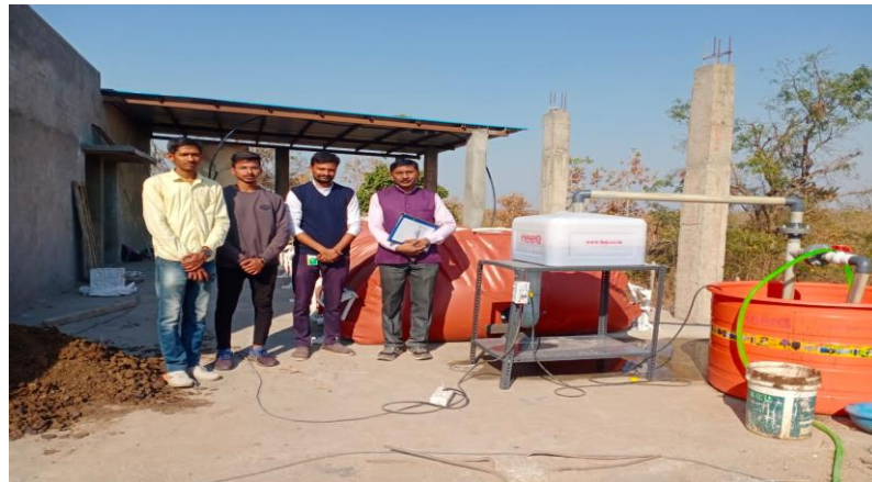
Fig. 9. Photo of actually installed plant
