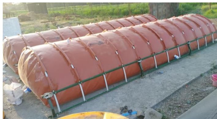
Fig. 7. Balloon-Type Digester
