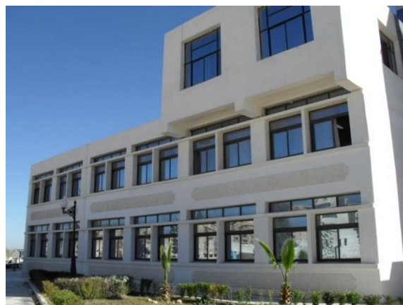
Fig.2. Facade of the Faculty of Psychology equipped with simple glazing « Stopsol Classic Bronze »
