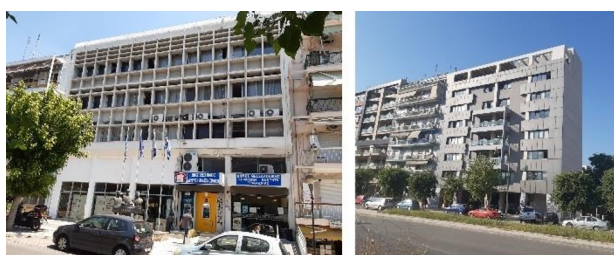
Fig. 2. The two case-study buildings. Left: Building A. Right: Building B.
