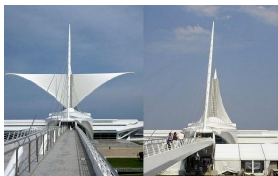
Fig.7. Milwaukee Art Museum with the brise -soleil opened and closed https://www.re-thinkingthefuture.com/case-studies/a3010-milwaukee-art-museum-by-santiago-calatrava-a-spectacular-kinetic-structure/ , access 30/7/2023.
