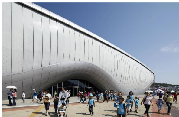
Fig.17. Cinematic facade of EXPO 2012-themed pavilion in Yeosu, South Korea. With closed slats, Architects: soma-architecture. https://transsolar.com/projects/one-ocean-pavillon-expo-2012 , access 09/2/2023
