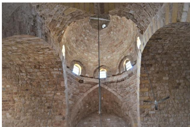
Fig. 1: View of the dome structure in Al Attar Mosque.
