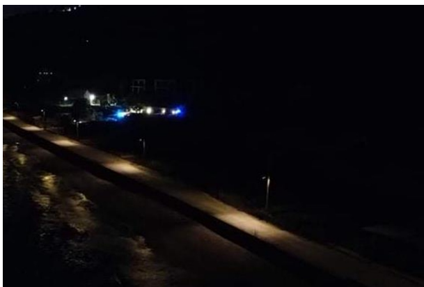
Fig. 7. New luminaires installed in Lourda beach along the sidewalk.
