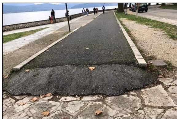
Fig. 4. The beginning of a part of cycling infrastructure lane.
