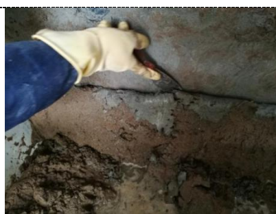
Figure 8. Expansion of grouting fluid in loose soil
