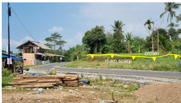
Fig. 5. Sarampad landslide shows the main scarp, crown, and road rebuilt in the depletion zone.
