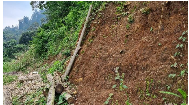
Fig. 1. Typical yellowish to dark brown residual soil and highly weathered breccia in the landslide area, exposed in the middle of the Cijedil Landslide (top) and in the crown area of Cugenang landslide (bottom).
