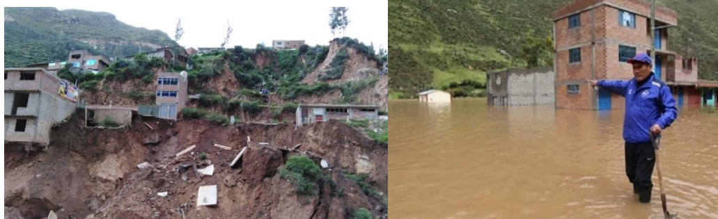
Fig. 2. Effects produced by El Niño 2019 in the construction zone of the Road
